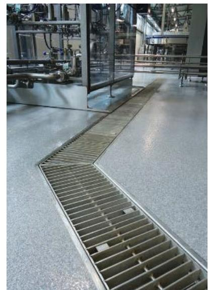
**Sv16H1: 16" WIDE STAINLESS STEEL TRENCH DRAIN WITH "V"-SHAPE BOTTOM & HORIZONTAL OUTLET**
