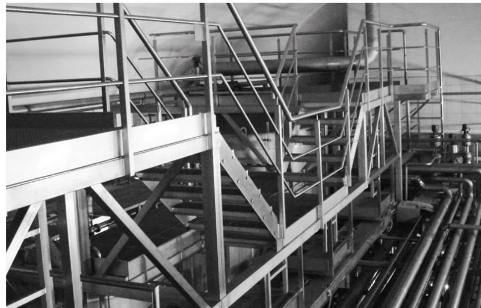
Technological platforms are elements of engineering structures that ensure safe access to a given industrial zone. Platforms are applied to eliminate hazards and ensure the safety of employees working at heights. Due to the customized shape of each platform, these constructions allow employees easy and safe access to specific working areas.
